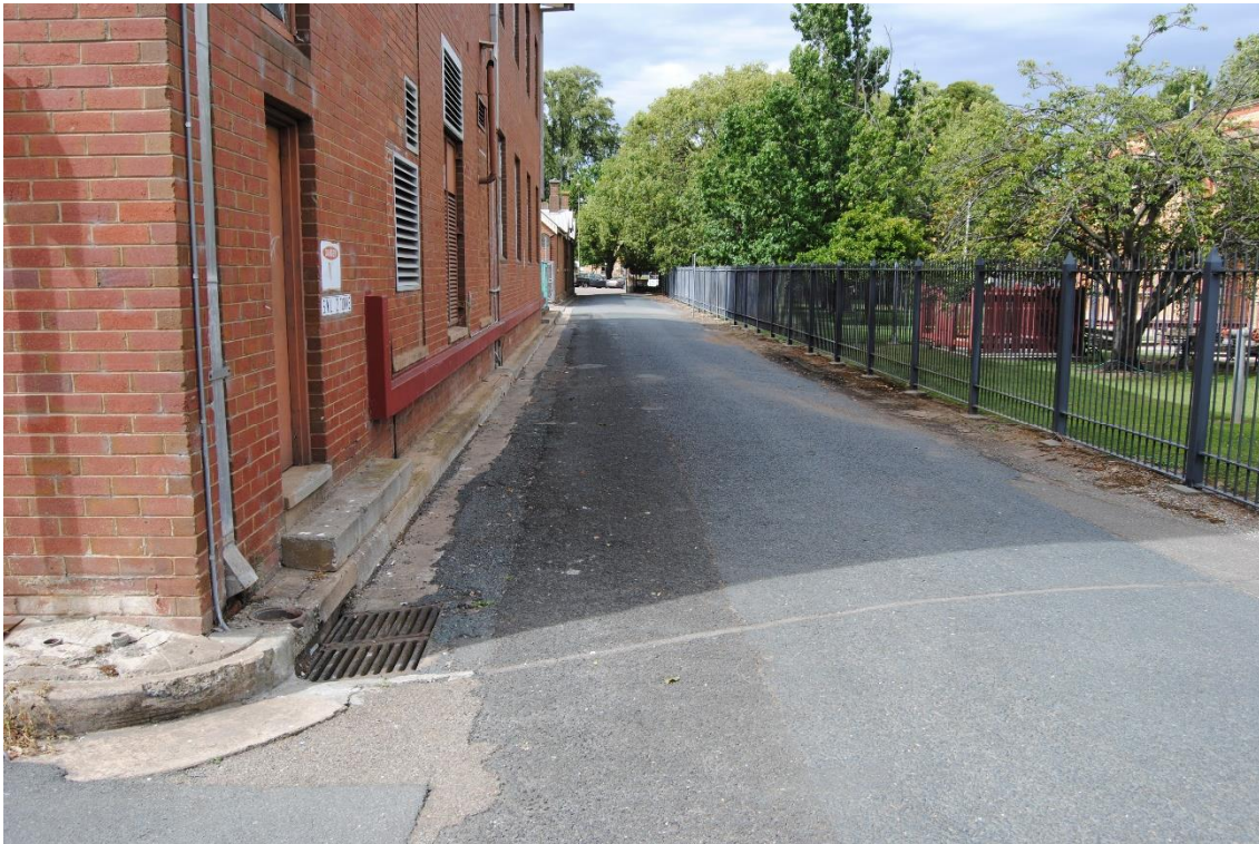
Figure 2. View from the lower northeastern end of Post Office Lane looking toward Montague Street with the existing grated inlet pit located at the entrance to the site in the foreground. A new grated inlet pit is proposed to be installed around the corner on the upslope side of the existing corner pit- in the extreme left hand side of the image.
