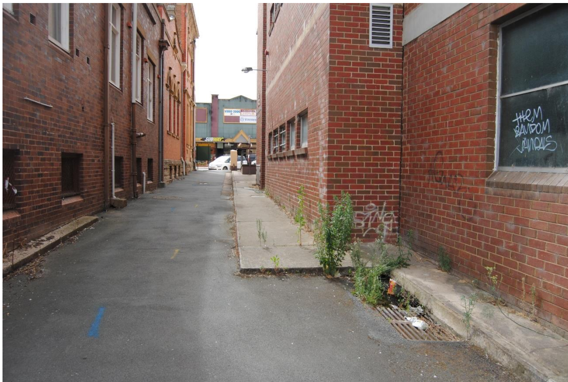
Figure 5. View of the existing grated inlet pit in the Post Office Lane at the front of the Telstra Exchange building and also showing the slope away from Auburn Street and from the edge of the subject site toward the pit.
